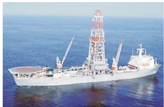
Drilling of Pasni X-2 well - 2005
